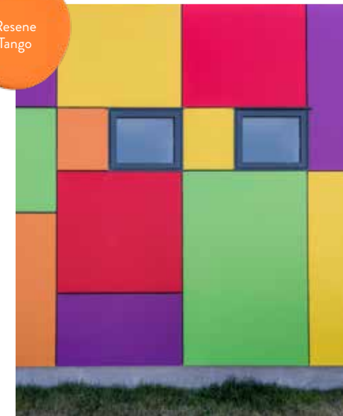
above: The candy-coloured façade of Hills Road Dairy won Richard's team a Resene Total Colour Exterior Maestro Award. The colours were inspired by a bag of Lollies Richard had purchased from the owner's previous dairy. This post-quake redesign was achieved using Resene Belladonna, Resene Wham, Resene Turbo, Resene Roadster and Resene Tango. Build by Horncastle Homes. Image by Stephen Goodenough.
