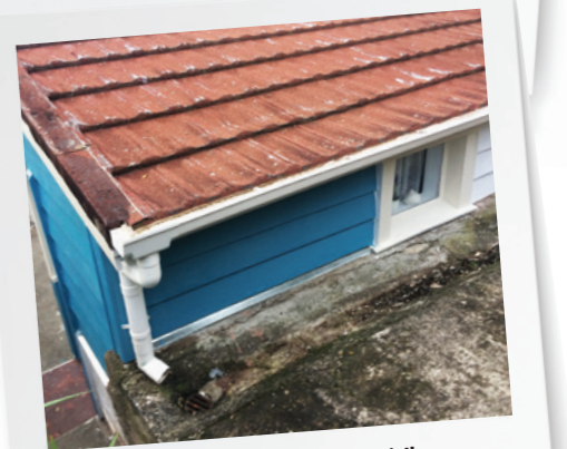
The red roof is still to be updated potentially using Zincolume.
