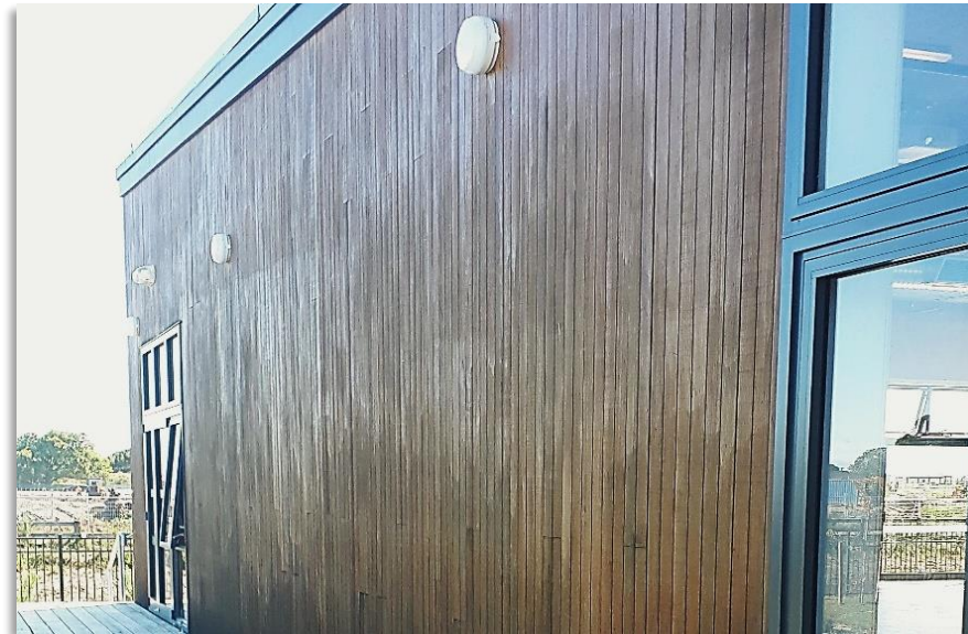
Colour affect – poor application / overlap
