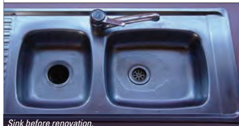
Sink before renovation.
